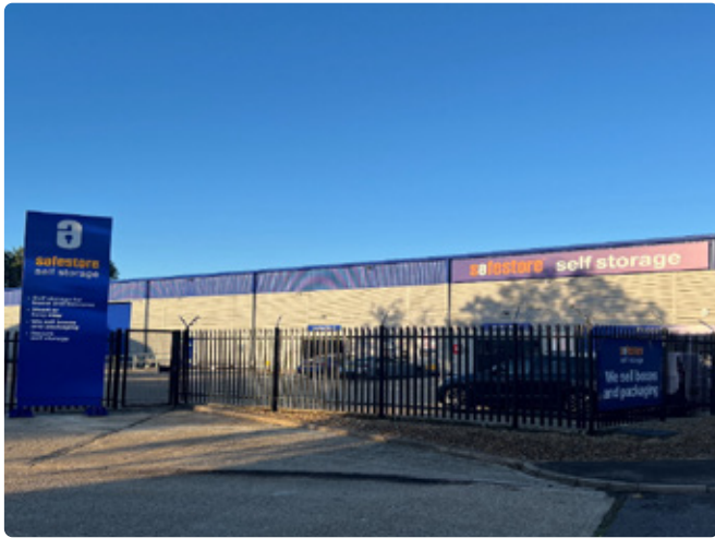
St. Albans – Existing building converted into a new Safestore.
