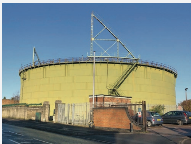
The last gas holder, just prior to demolition
