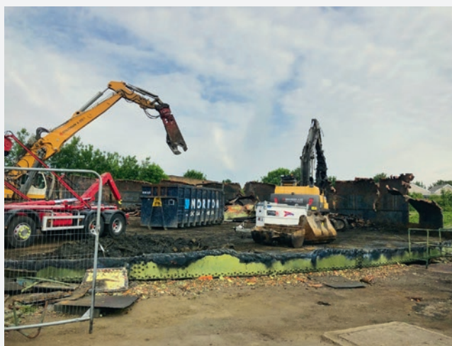
During the final stages of demolition
