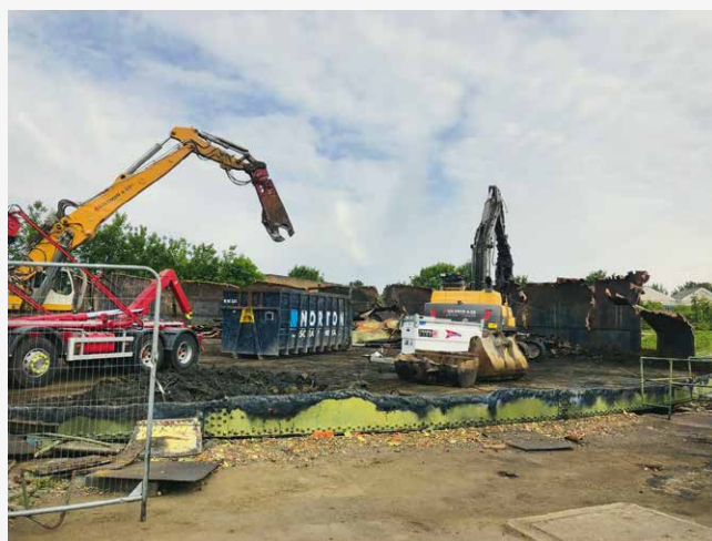
During the final stages of demolition
